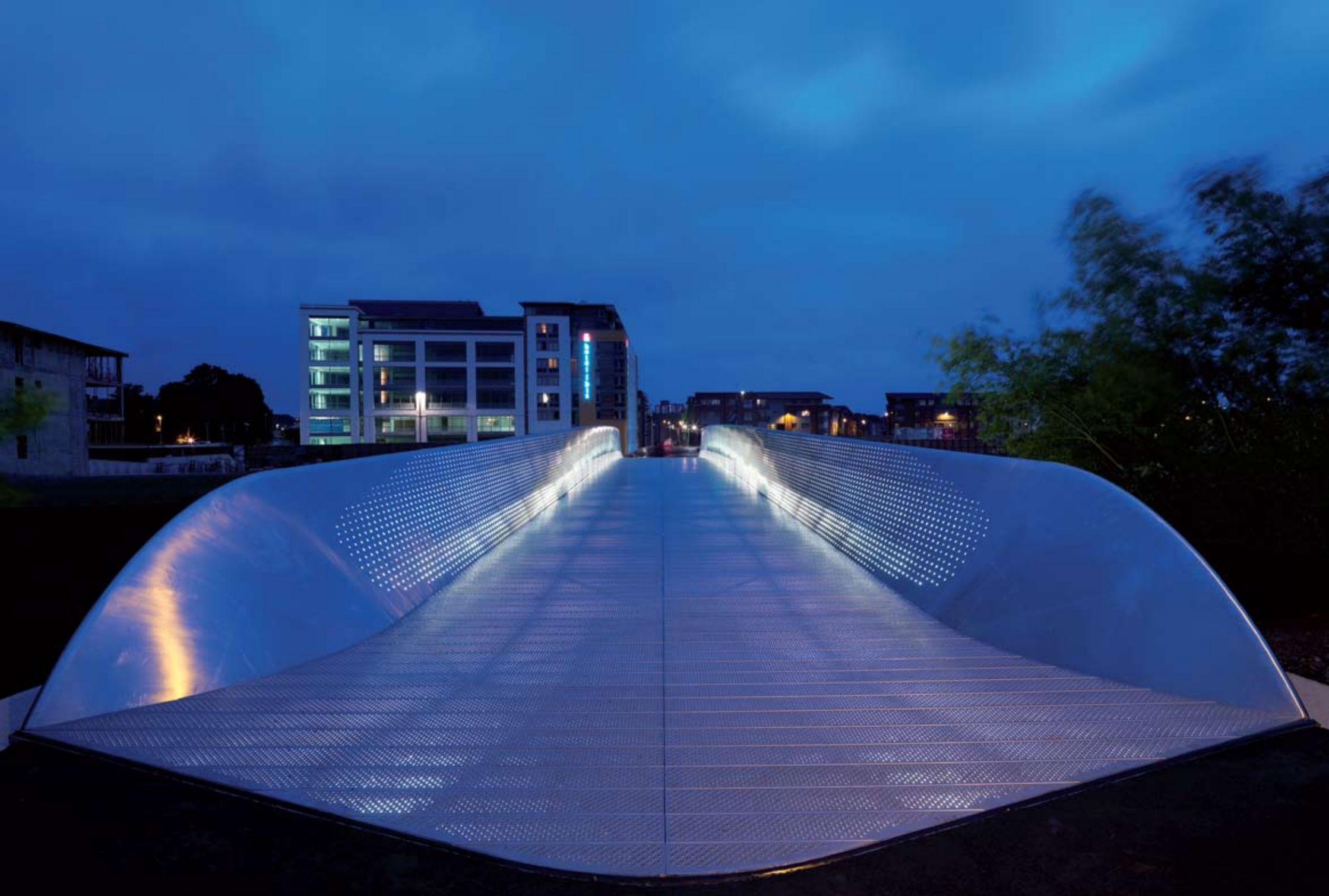
The completed structure
