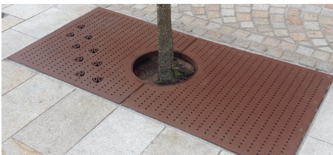
Bespoke tree grilles with intricate laser cut designs
