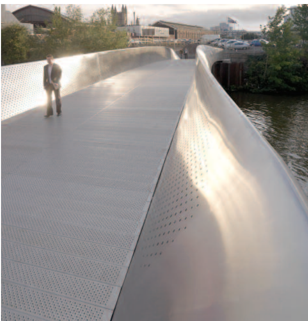
The 55m Meads Reach duplex bridge at Temple Quay, Bristol
