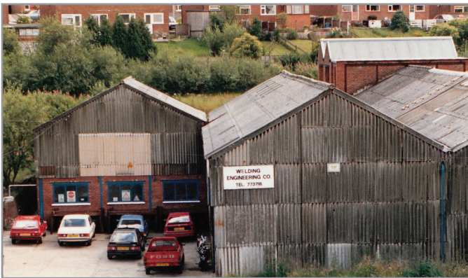
The Group's second site at Cranberry Lane, Darwen
