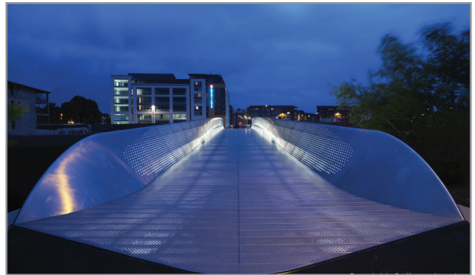
Mead's Reach Bridge, Bristol, fabricated by m-tec, our division which specialises in stainless steel architectural pieces
