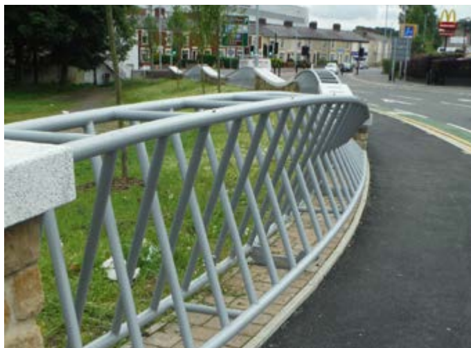
Speciality railings for the new Ewood Gyrary System in Blackburn
